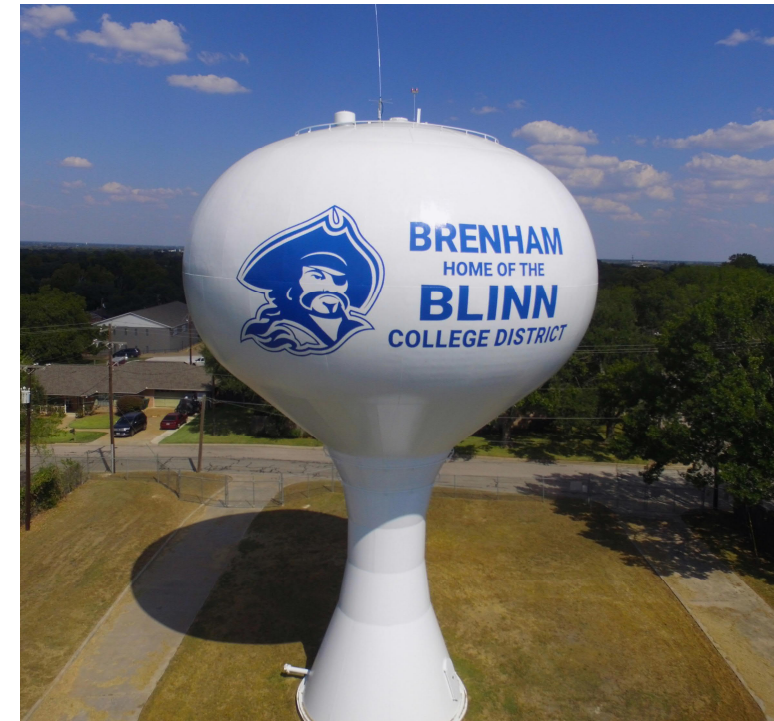
Atlow Elevated Storage Tank
