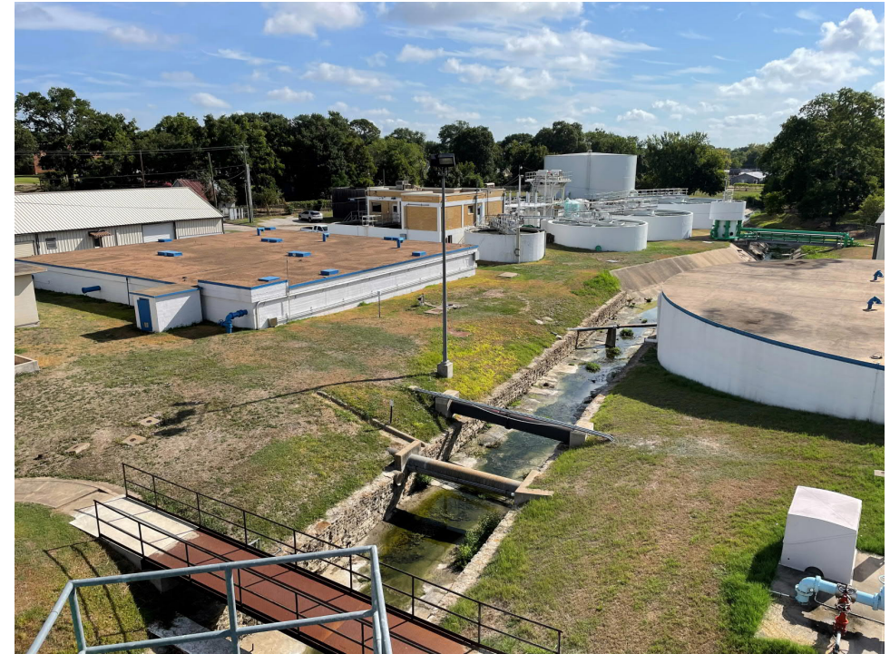
Surface Water Treatment Plant
