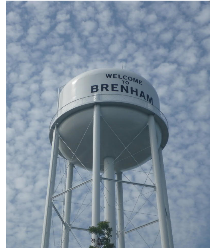
Church Street Elevated Storage Tank
